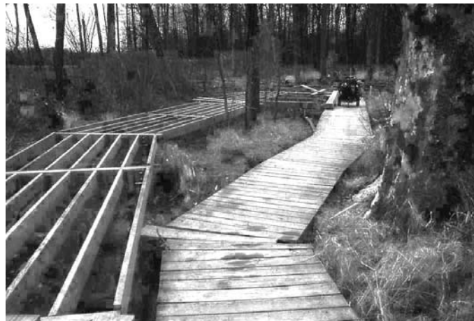
New Boardwalk Being Build Adjacent to Old
